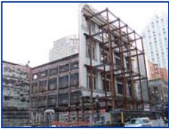
A new building is erected within the shell of the old
