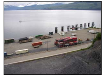
Tideland fill for new Hoonah Marine Industrial Center
