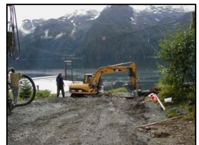
Tank farm and utility upgrades being installed in Pelican
